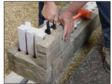
Diagram 22—Wall end example
