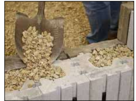
Diagram 5—Fill cores with free draining aggregate
