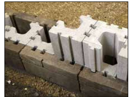
Diagram 21—Second course construction
