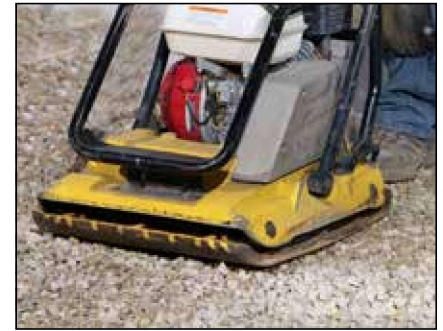
Diagram 18—Leveling Pad
