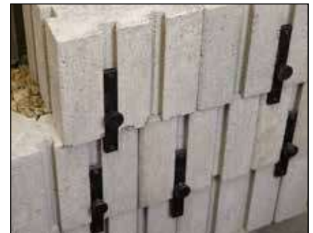
Diagram 6—Lock connector to the block in front
