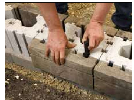
Diagram 20—Placing veneers onto modular block
