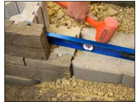
Diagram 7—Stepping up the base
