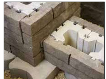
Diagram 23—Ending a wall at a column example
