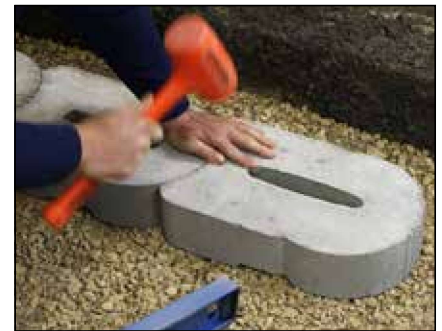
Diagram 3—Lay and level base block
