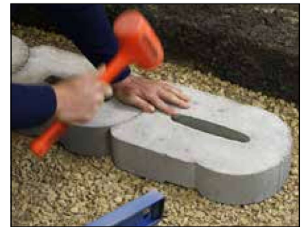
Diagram 19—Lay and level base block
